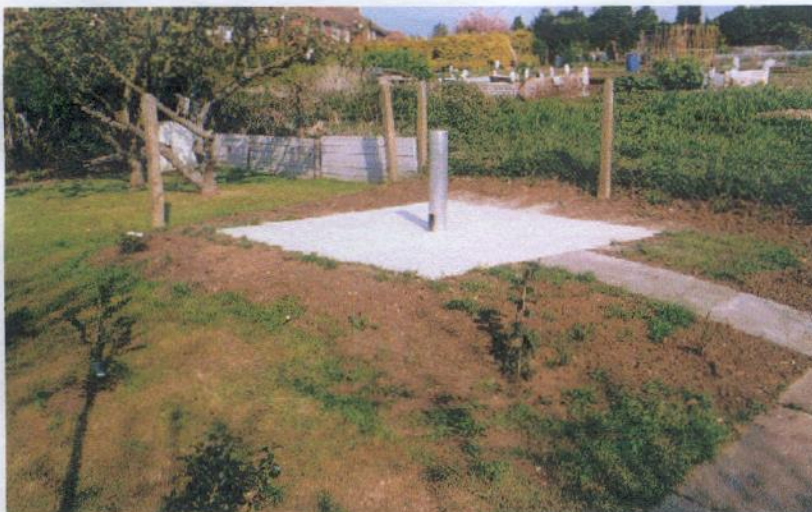
The completed base
