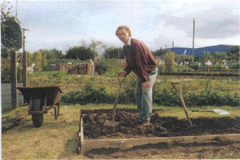
Digging out the base
