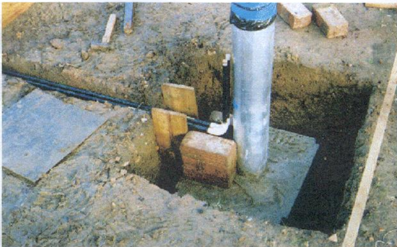
Installing two plastic conduit pipes
