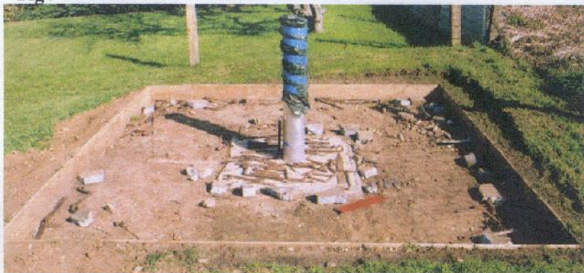
Completed Pier foundation
