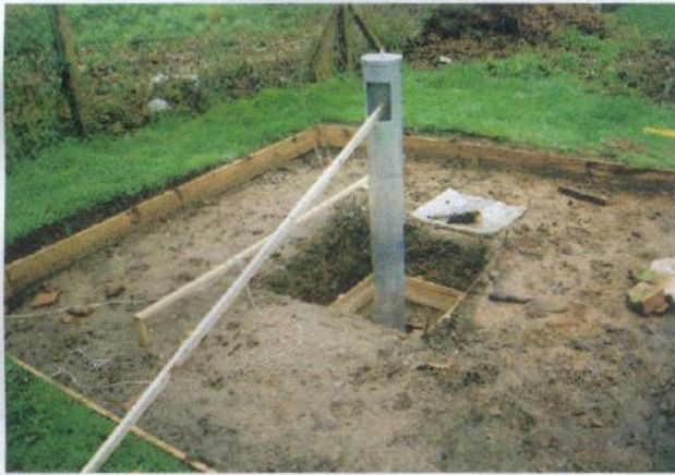
Supporting the pier before concreting in
