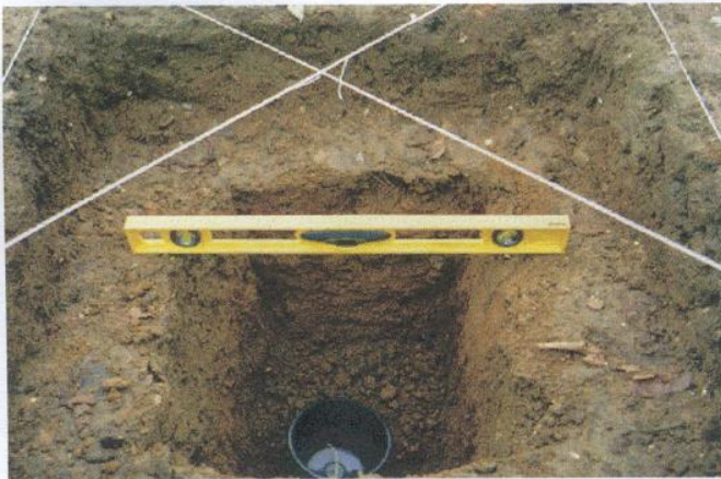
The pier hole
