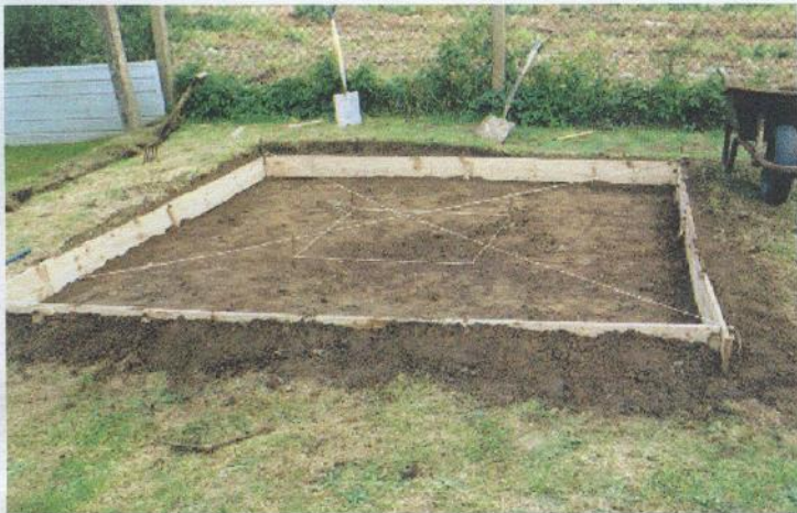
Marking out the hole for telescope pier
