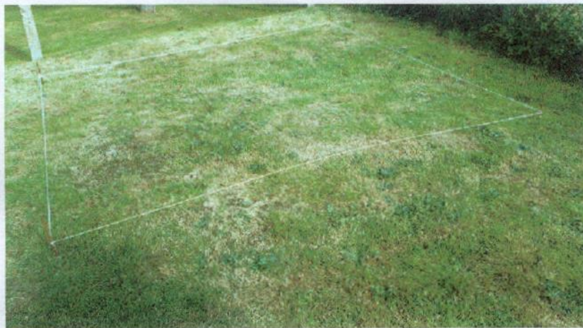
Marking out the observatory base
