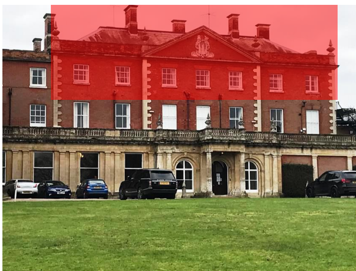
Image showing area affected by the flames (Bill Barton)
